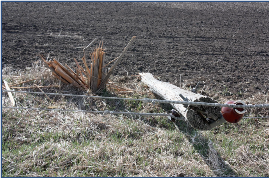
LEFT: A pole lies on the ground south of Ferney after a disc operator working a farm field hit it and broke it off in April.
