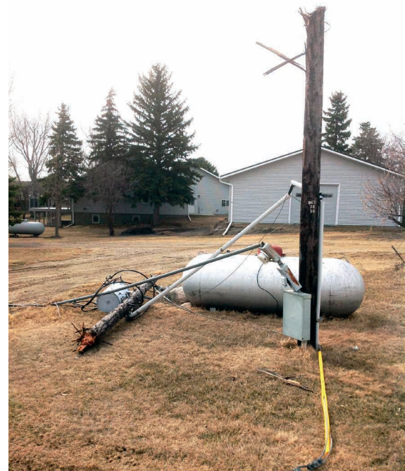
ABOVE: A pole, meter, and transformer broke near Mina Lake in March after a commercial truck hit the guy wire supporting the pole.
