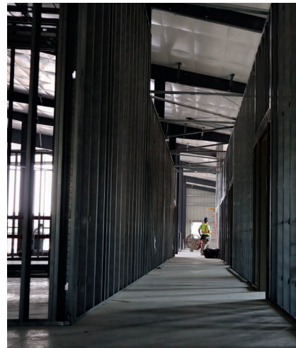
The framing for the interior walls are being installed.
