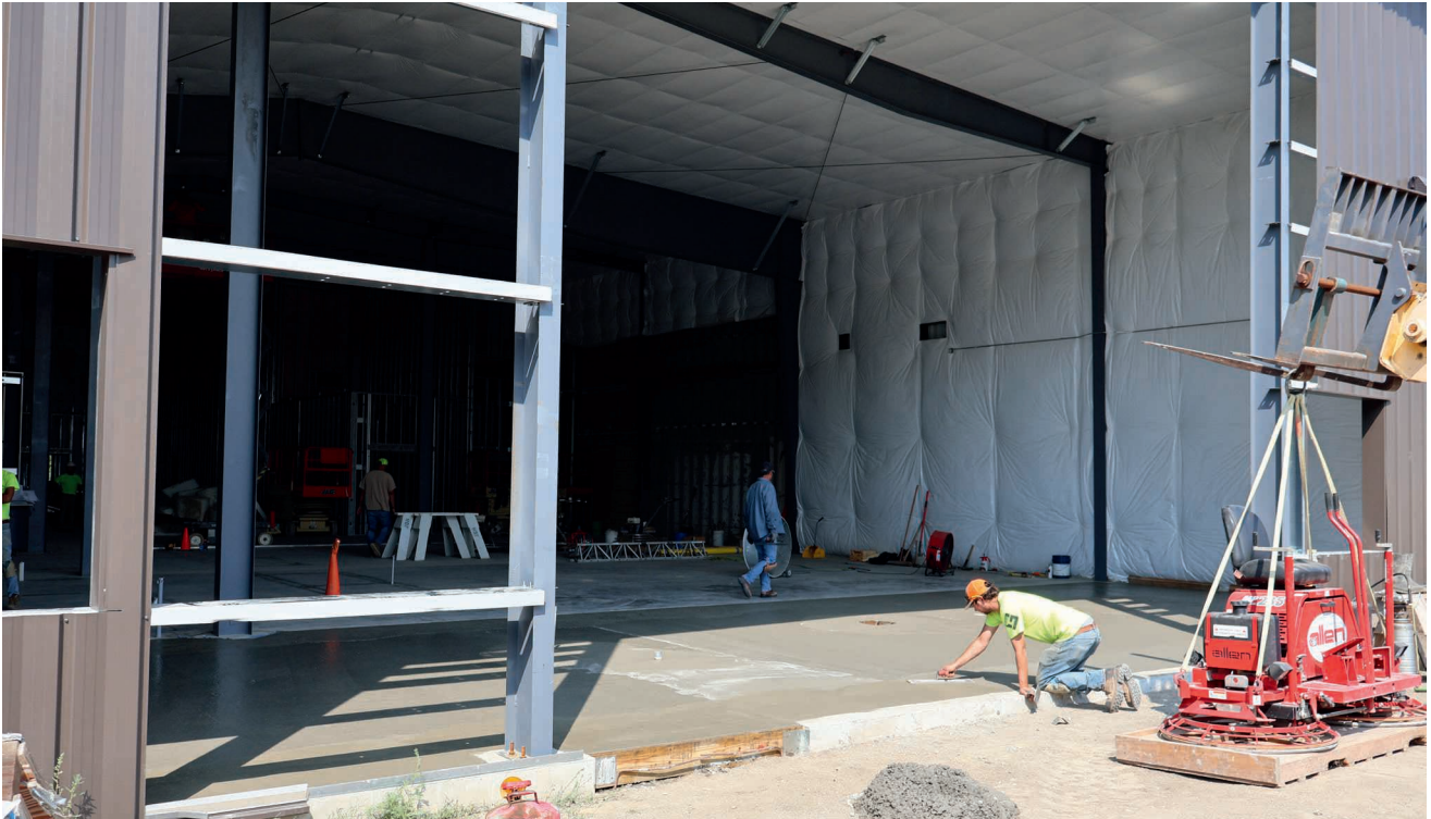
A construction worker smooths the final pour as other workers put up the steel beams for the walls.
