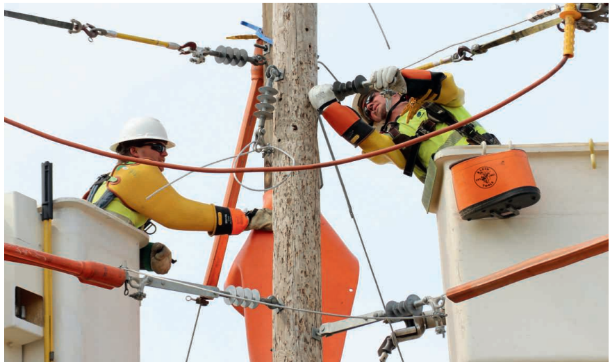
MTC is a prime training ground for future co-op linemen. Photo by Billy Gibson
