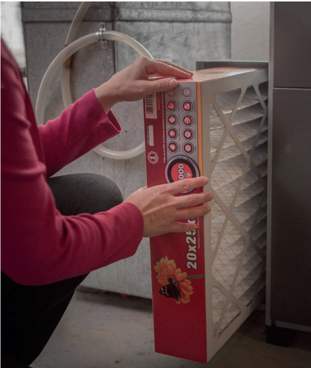
Replacing the filter on a heating and cooling system every month will keep it running at peak efficiency.
