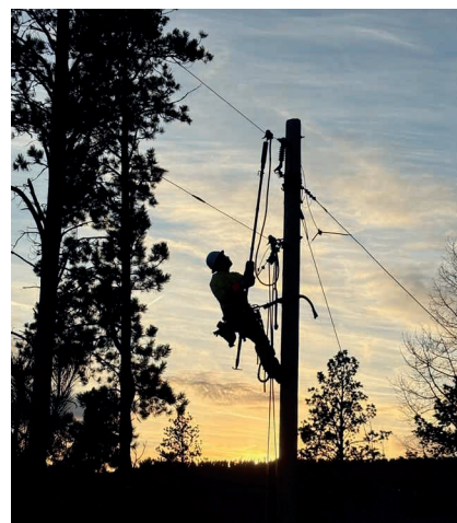
An assisting lineman from West River Electric Cooperative installs a ground on the line to be further worked on.
