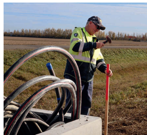
Tyler pounds in a stake to mark where underground cable will go.
