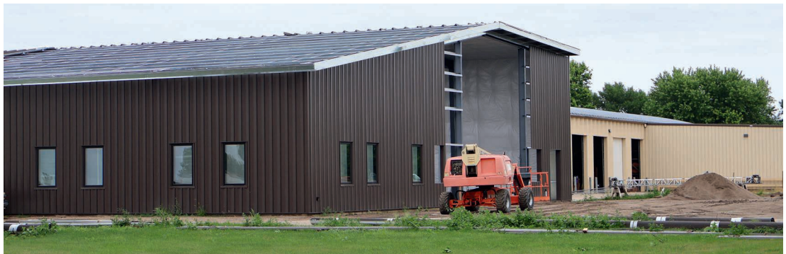
The east side of the building is open, allowing access during construction.
